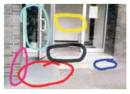
**Red:** Inclination of the ramp is not 12:1
