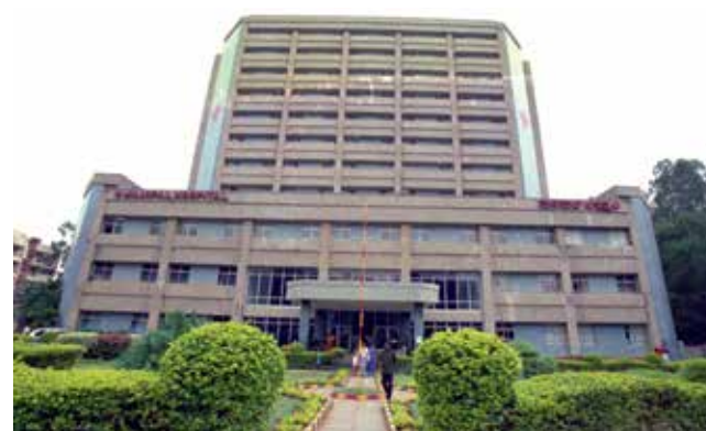
Manipal Hospital, Bengaluru
